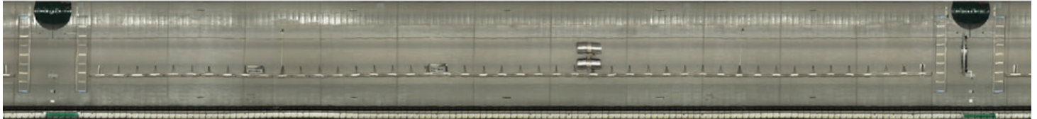
Cylindrical orthophotography of a road tunnel
