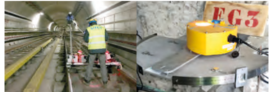
Railways tunnel ScanTubes® survey.
