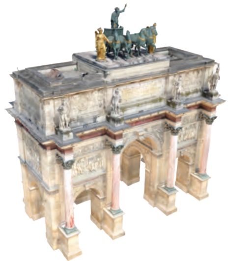
3D digital twin of the "Arc du Carrousel du Louvre", based on photogrammetric surveys to enable a structural health monitoring.
