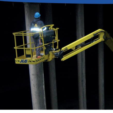
VERAO® is an application developed by SITES which enables the inspections of structures or parts of structures according to the client's points of reference (nature of visits, plan...). This tool enables you, as early as the field study, to map the disturbances observed via a PC tablet whilst also generating a detailed database.
